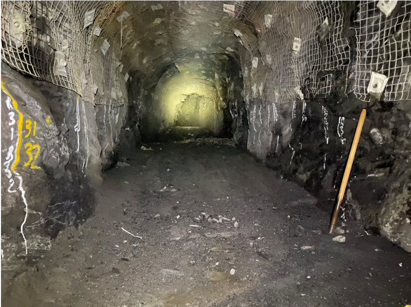
Fig.3 Golden Eagle Underground - Development Drive
