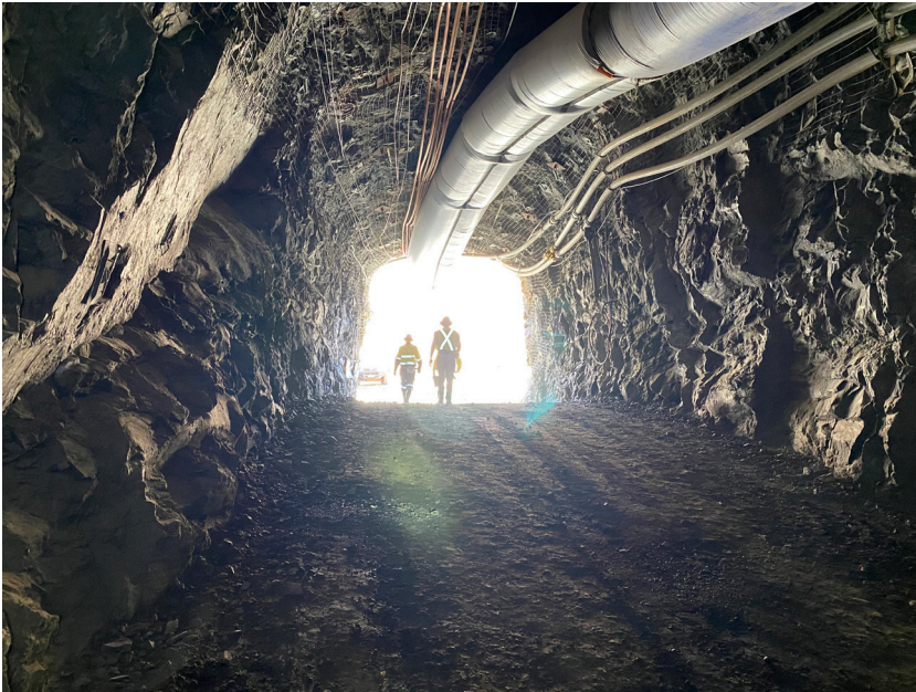
Fig.2 Golden Eagle Underground Portal
